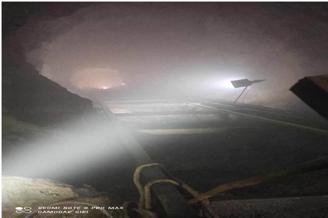
Figure: Inclined tunnel channel fixing
