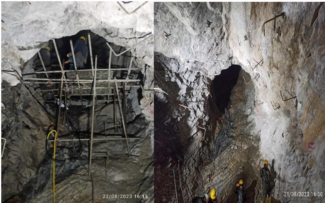
Figure Dowel bar installation at lower bend
