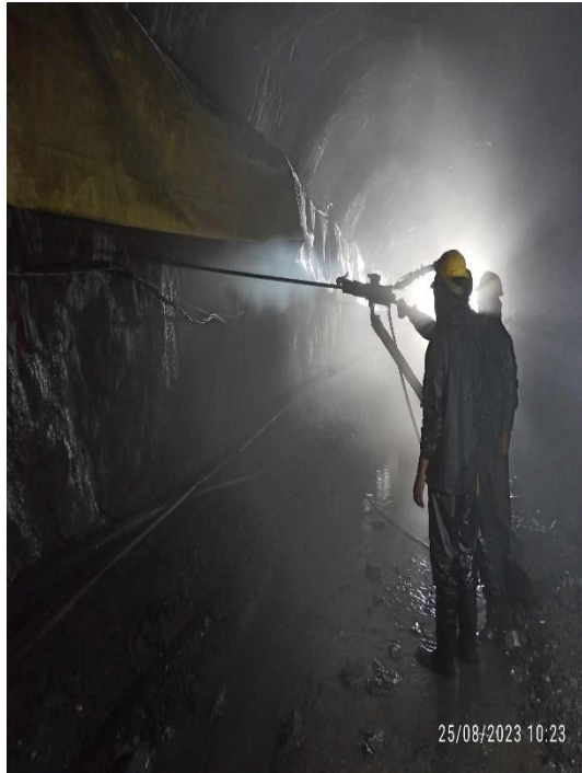
Figure Rock Bolt Drilling at Upstream Face 2
