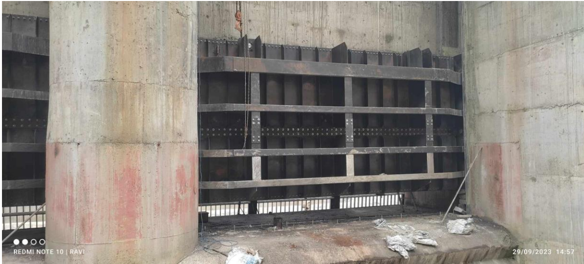
Figure undersluice gate
