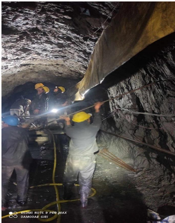
Figure: Rock bolts drilling at face 2
