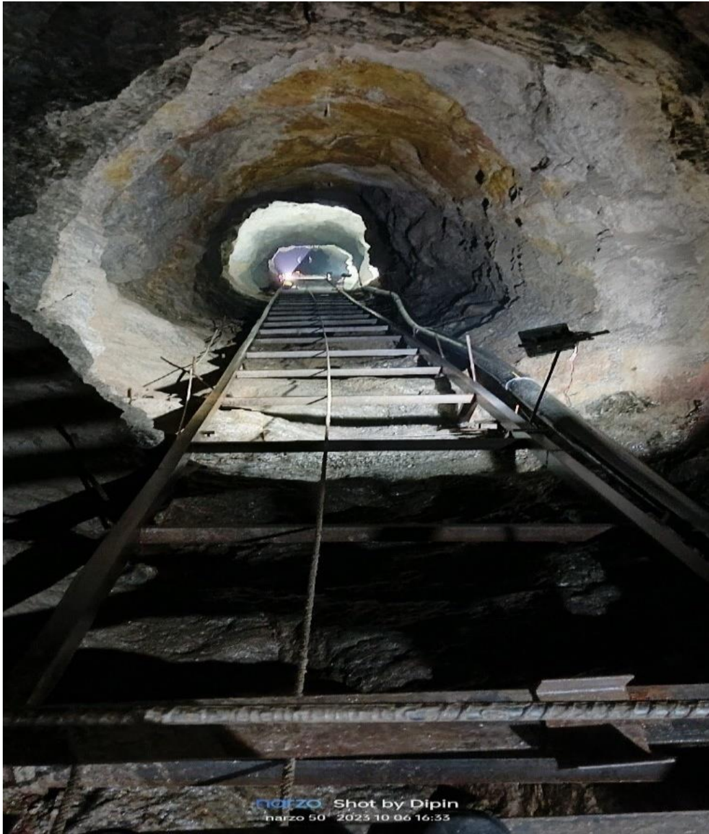
Figure: Image of installation of rail line at inclined tunnel section
