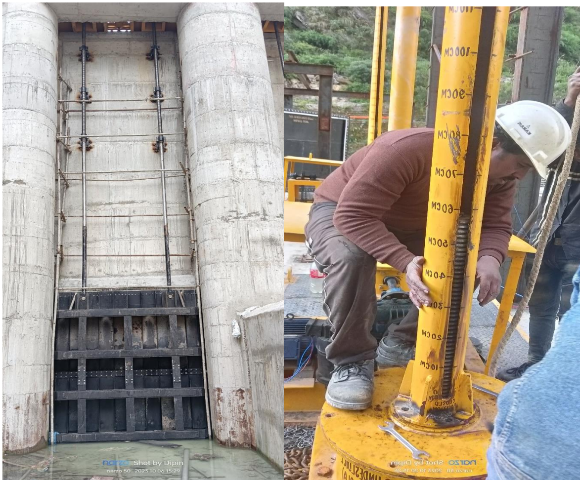
Figure: Assembly of motorized screw hoist with undersluice stoplog gate
