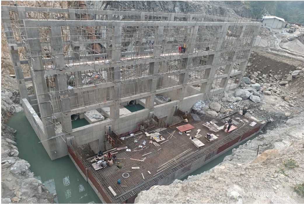
Figure :Rebar work in tailrace pool
