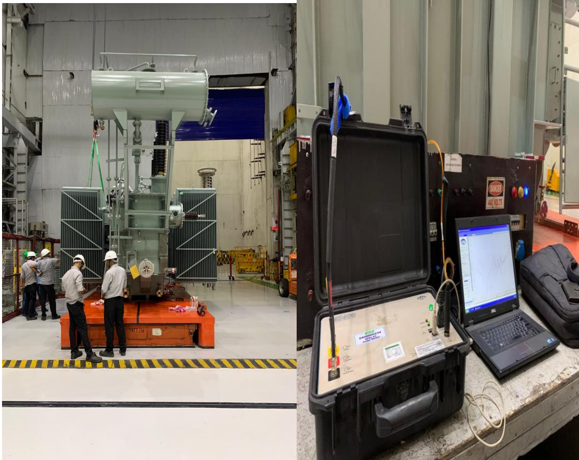
Figure Complete assembly of power transformer
