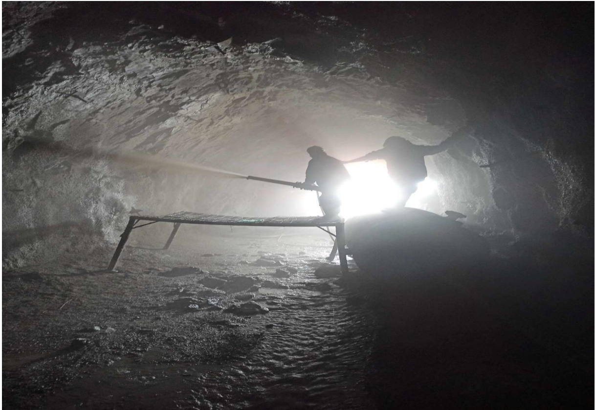
Figure Shotcrete works at HPS
