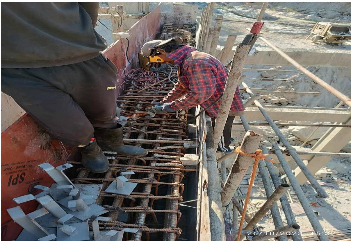
Figure: Embedded parts installation in tailrace
