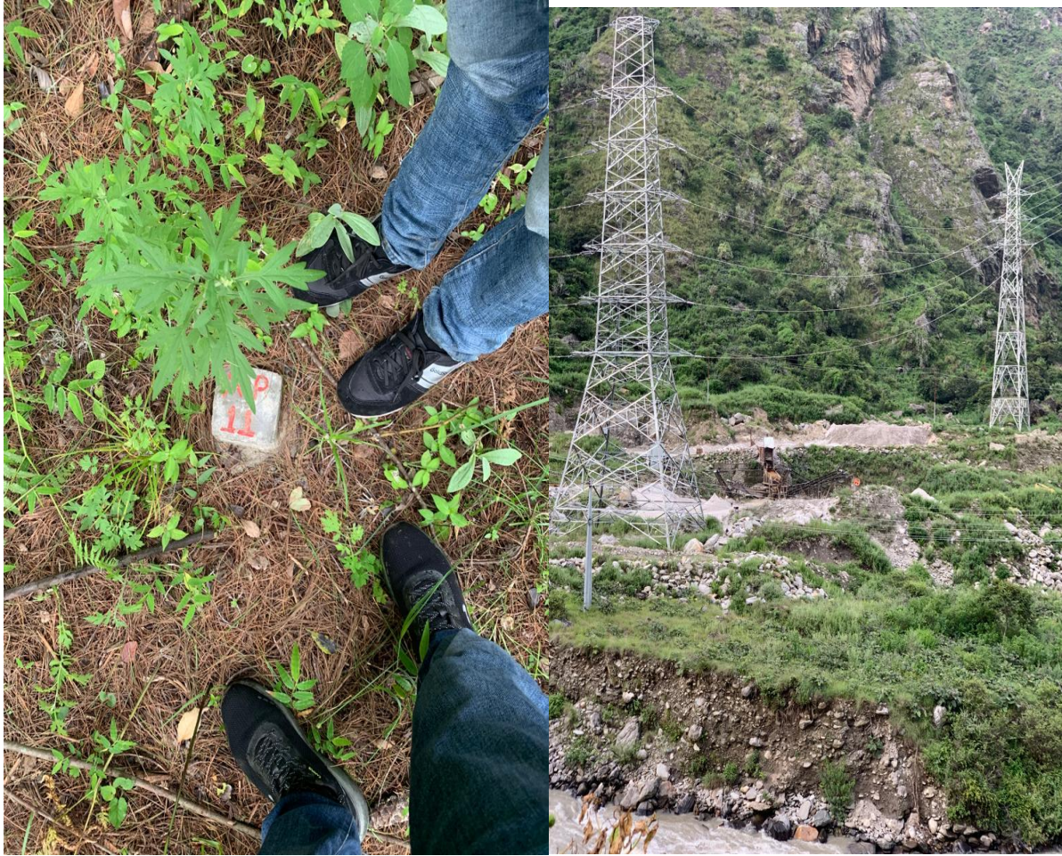
Figure Check Survey along the alignment of transmission line
