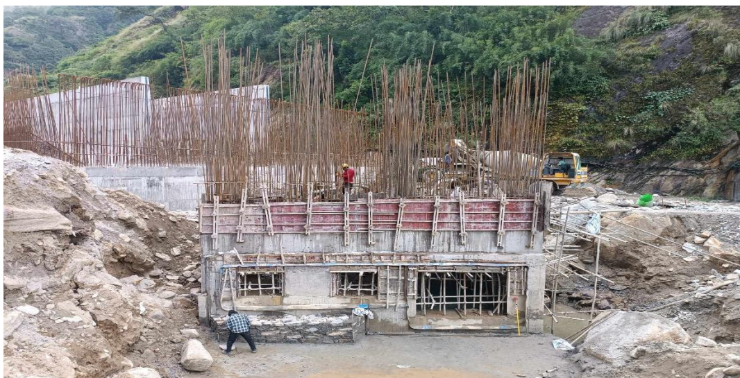
Figure Concreting at sand flushing
